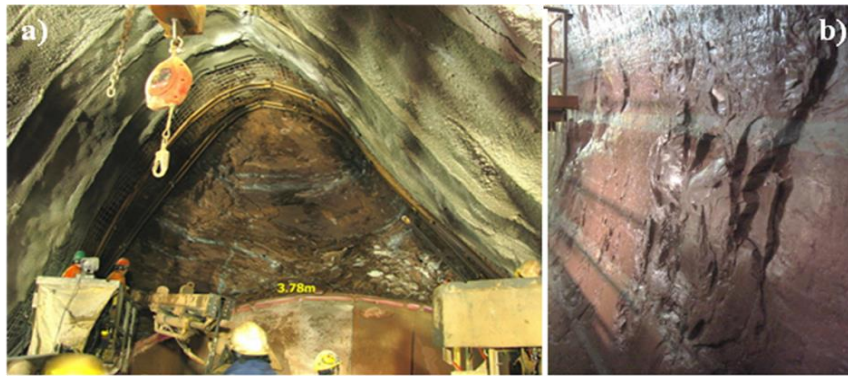
Figure 2: Observed failure in the Queenston in Zone 4, showing a) typical large notch formed in the high stress regime and b) minor sidewall spalling not associated with structural features.
