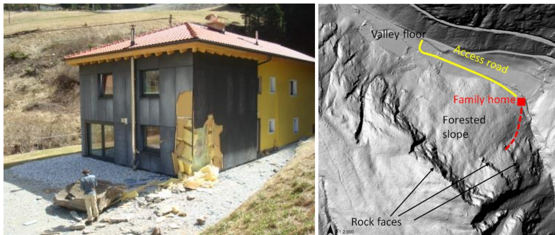
Figure 1: Family home on the foot of the slope damaged by the rock-fall 2011, situation sketch.
