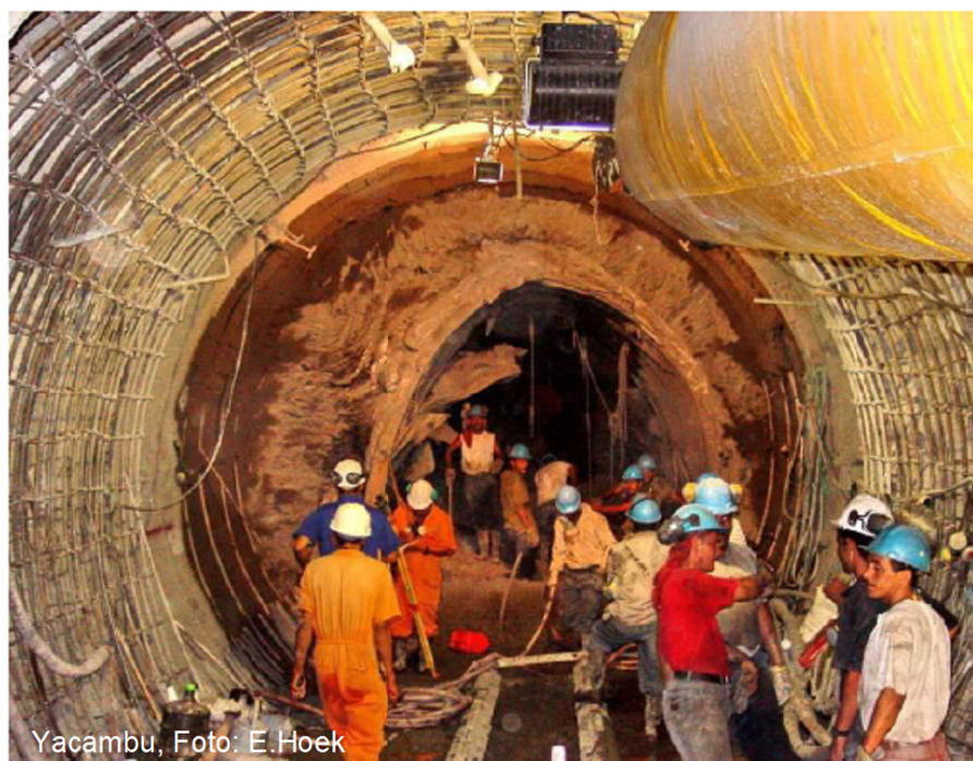
Figure 2. Reprofiting works in the Yacambu adit. Please note the basically completely destroyed initial support ahead of the current advance.
