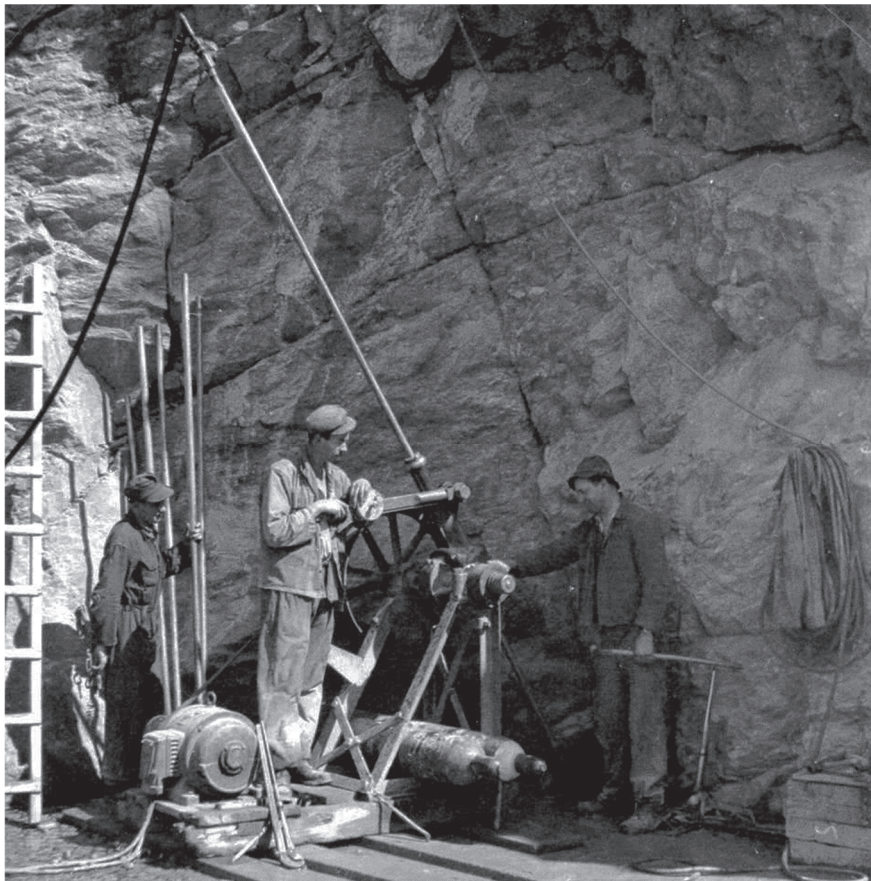
Figure 1. Grouting work in pioneering days: Exploratory drilling at Kaprun HPP, CRAELIUS CX 42 drill, INSOND (1950)
